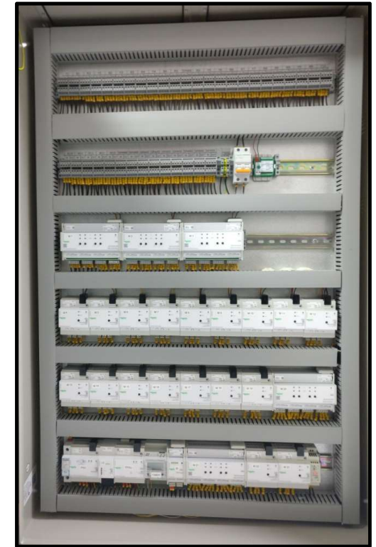
Typical Lighting Control Panel ( LCP)
