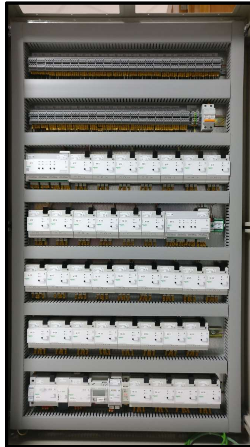
Typical Lighting Control Panel ( LCP)
